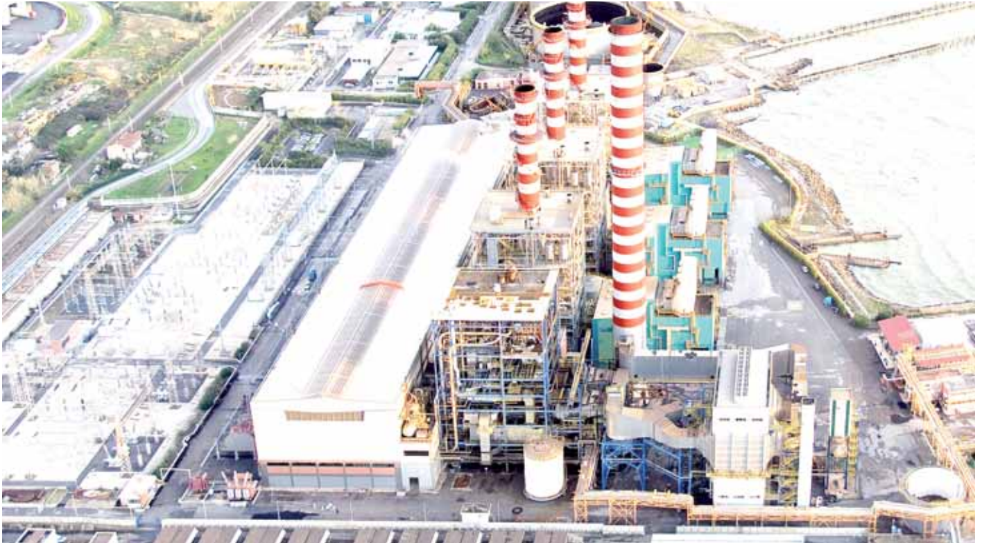
A power generation plant
