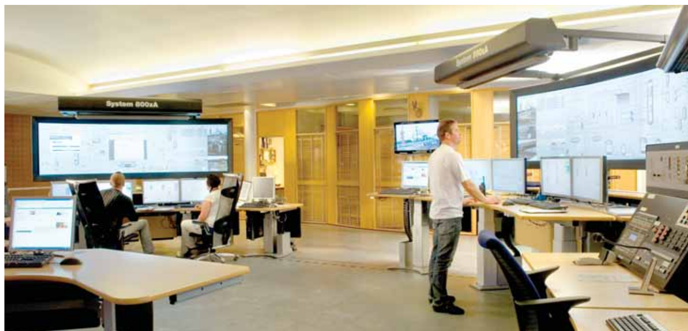
Control room using 800xA platform
