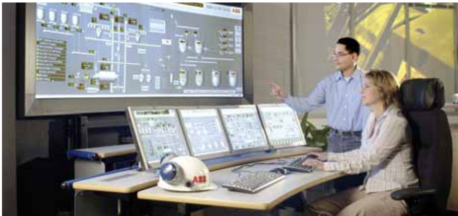
Control system operator workplace
