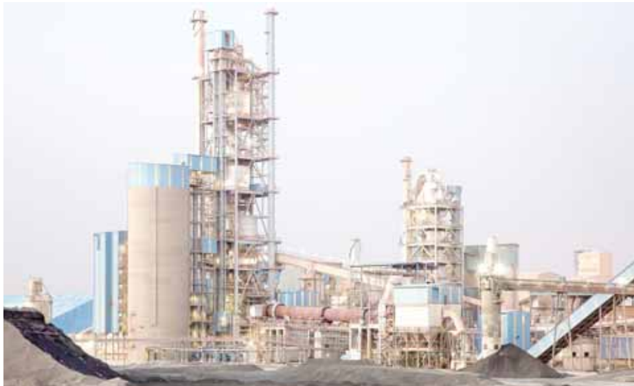
Total cement plant view
