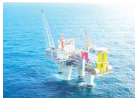
An offshore platform
