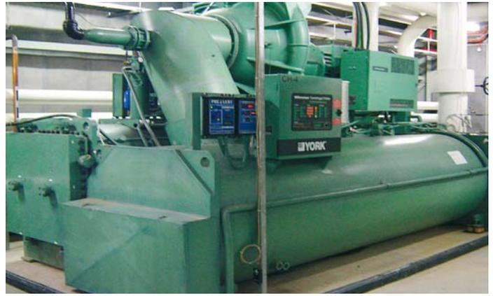
Throttling valves on the water-cooled chillers have been replaced with variable speed drives.
