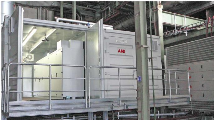
The water-cooled ACS 1000 medium voltage AC drives were installed ready for connection in special, fully air-conditioned containers.
