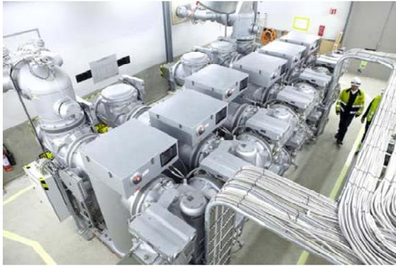
installation has been reduced to about one-fifth of the size of a traditional air-insulated substation.
