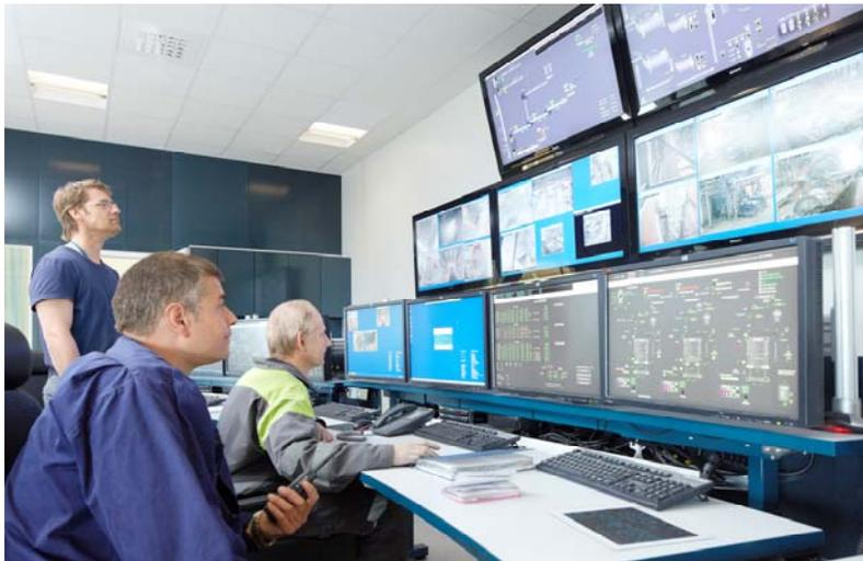
The entire site process at Aitik – including the concentrator plant, conveyor systems, pumping stations and even the mine's own sewage plant – is controlled by ABB's Extended Automation System 800xA. This is more than a DCS: It is a platform by which to integrate a diverse assortment of equipment, systems and applications to provide a common visual interface.
