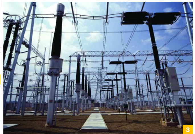
1 Pulling the Gotland DC cables ashore in the 1950s. 2 An ABB engineer on site in Gotland. 3 In a large HVDC station, it must be possible to isolate the power circuit. This is done in the AC switchyard with help of instrument transformers and 500kV circuit breakers.
