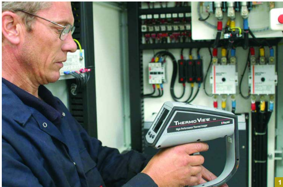
1 Thermal imaging is used to inspect cables and unenclosed low voltage switchgear. Being a non-contact technique it is ideal for situations where downtime needs to be avoided.
