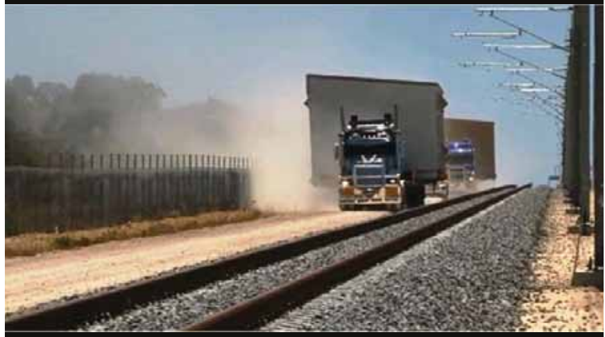
This clips shows how the team triumphs over logistical challenges during the Butler Extension Project Feeder Station Installation
