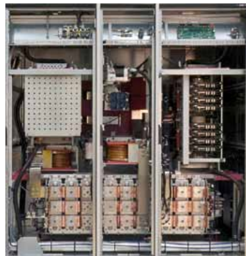
Phase converter unit of the water-cooled ACS 5000
